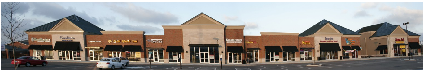
Martinizing Dry Cleaning at West Chester Village Retail Center By Elford Development
