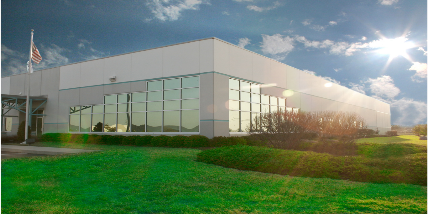
Rite Track Equipment Services Union Centre Boulevard District
