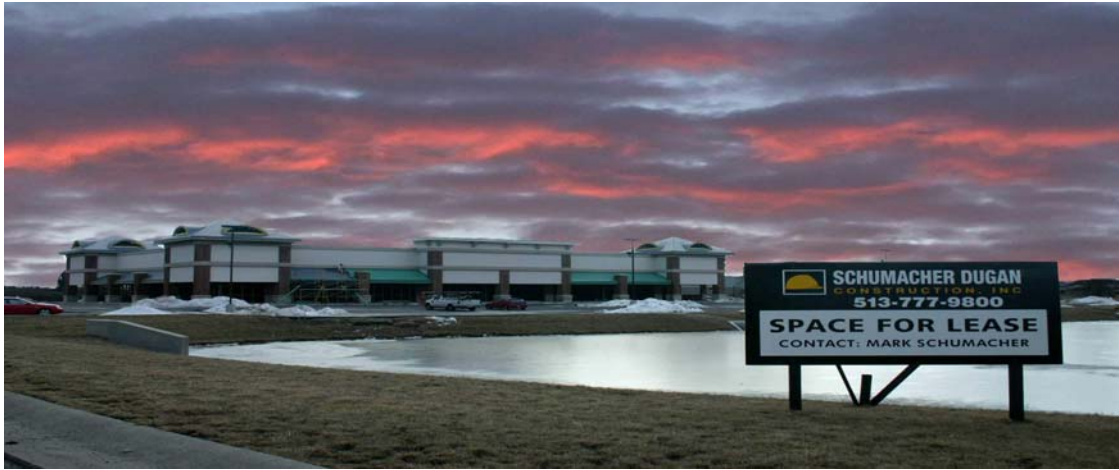
State Farm Insurance at Union Centre Retail Plaza Developed by Schumacher -Dugan Construction Company
